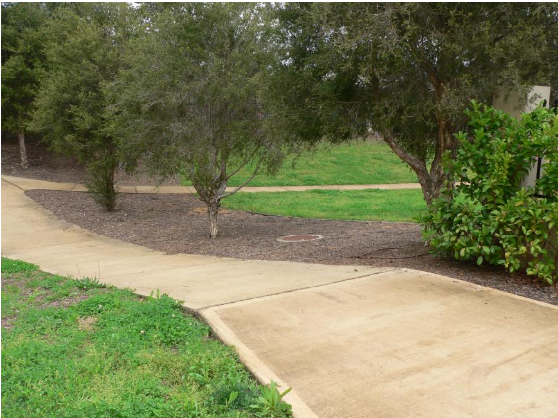
Plate 4: Levee Option 1 - View of the eastern end of the drainage reserve between approximate Ch. 30m and Ch.60m on the levee alignment.
