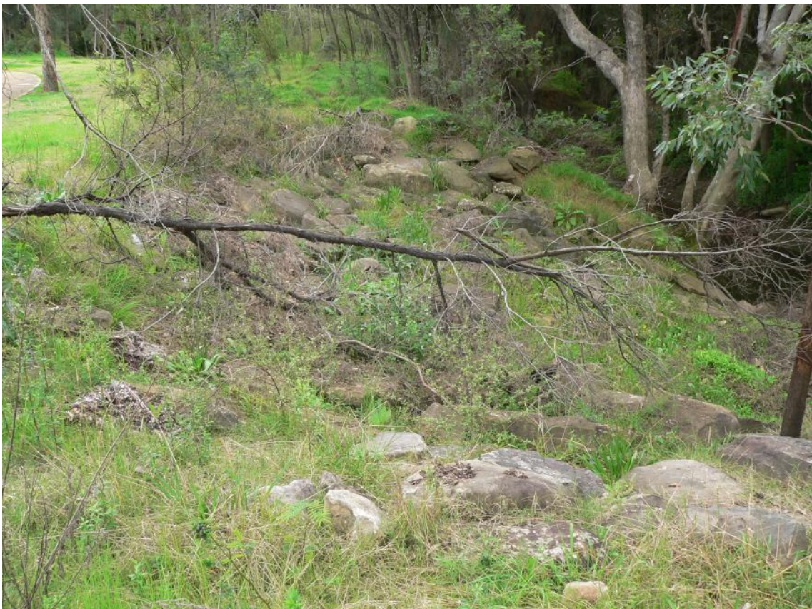
Plate 8: Levee Option 1 - View of boulder lined upper slope at approximate Ch. 80m on the alignment. The levee at this location will be a concrete wall.
