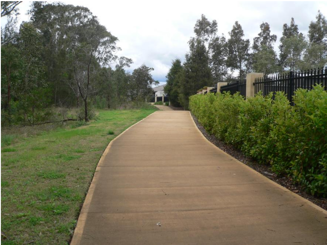
Plate 2: Levee Option 1 - Another view of similar site conditions at the rear of the properties.
