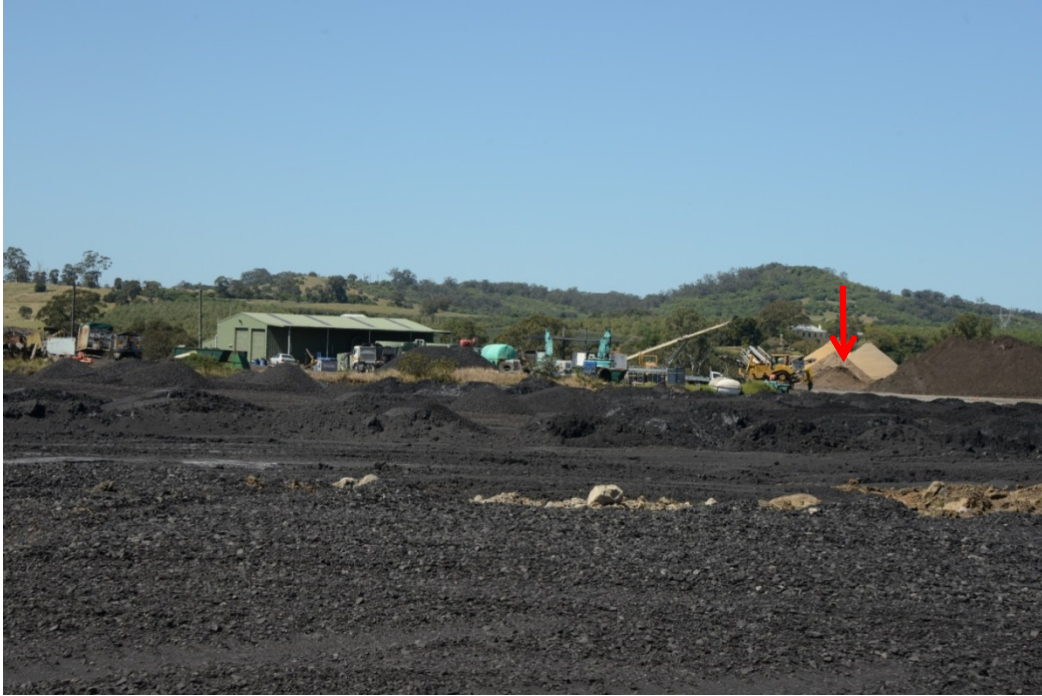
Figure 19 View from coal washery across Camden Soil Mix site to 'Glenlee', with the house (arrowed) visible immediately to the left of the light-coloured mounds of soil. (Photo: C Betteridge, 27 September 2013)
