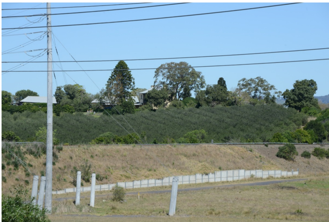
Figure 18 Telephoto image from south-east part of the Study Area to 'Glenlee', showing main Southern Railway line across centre of photo, with the house and garden beyond and part of the olive plantation on the slopes to the west of the house. (Photo: C Betteridge, 27 September 2013)
