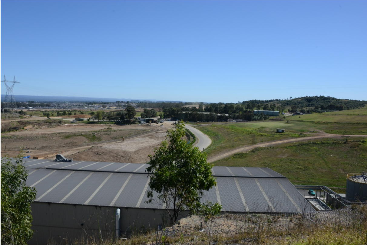
Figure 24 View looking west and north-west over the Recovery Park site. (Photo: C Betteridge, 27 September 2013)
