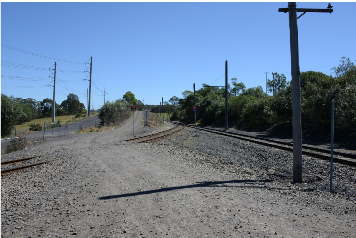
Figure 14 View north-west into Glenlee Precinct, showing western end of the 'Y' of the private rail line spur into the site from the main Southern Railway Line. (Photo: C Betteridge, 27 September 2013)
