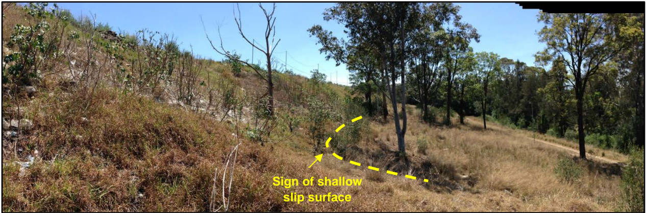
Plate 6: Eastern Embankment – a localised section near the Northern end
