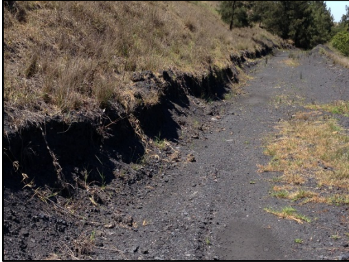
Plate 2: Close up view of existing erosion scarps
