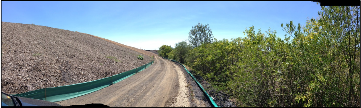
Plate 5: General View of the Eastern Embankment - taken from the Southern end
