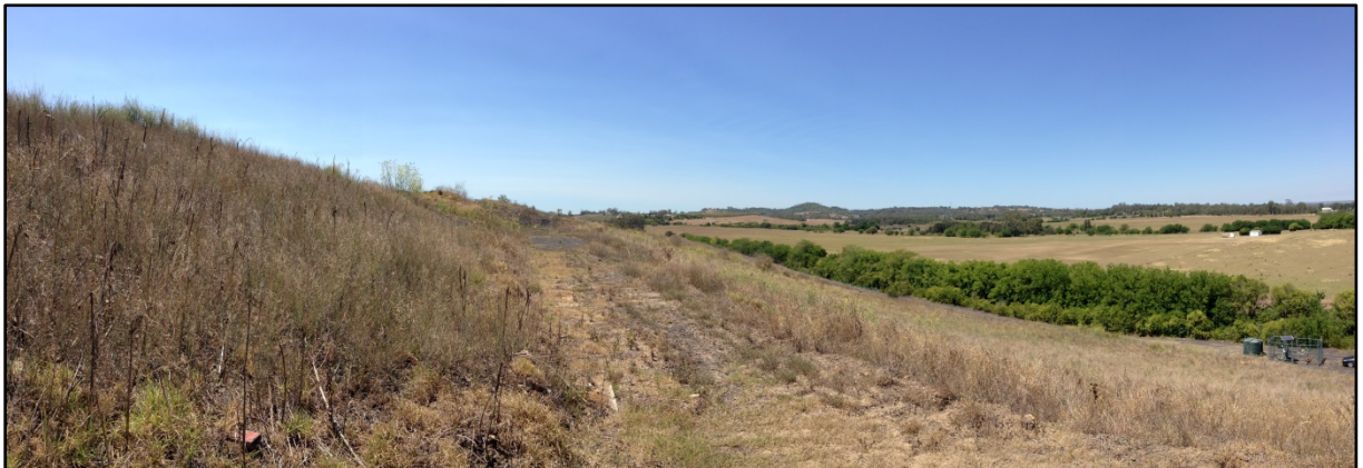
Plate 3: General View of the Southern Embankment – Upper Bench
