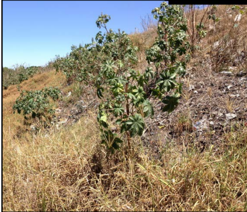
Plate 7: Eastern Embankment - Close up view of the embankment surface materials - taken at the Northern end
