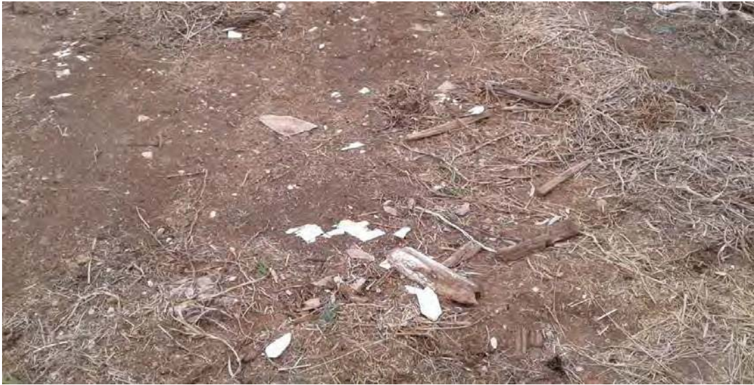
Photograph 5 - Fragments of fibrous cement material in the immediate vicinity of stockpile in central northern portion of site.
