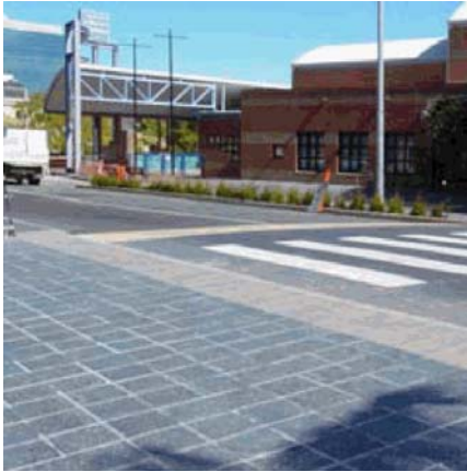
Stonevue paver thresholds with asphalt top and concrete ramps
