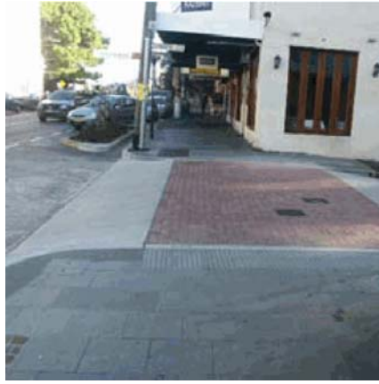
Stonevue paver top and concrete ramps
