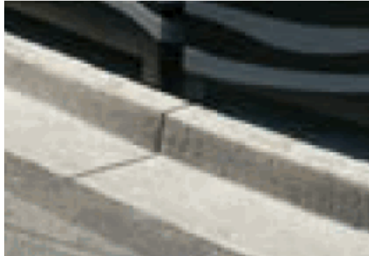
Standard Concrete kerb & gutter
