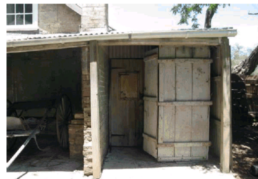
Figure 4.15 View showing brick and timber addition to the northeastern corner of the building.
