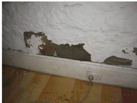
Figure 4.6 Damage caused by rising damp in the c1810 building.
