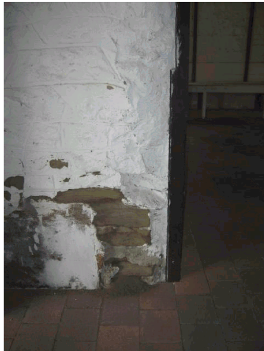
Figure 4.19 View of deterioration to stonework due to rising damp and delamination.
