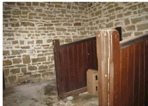
Figure 4.13 View of ground floor of stables—note the damp areas to the concrete floor and the boring activity in the front timber post.
