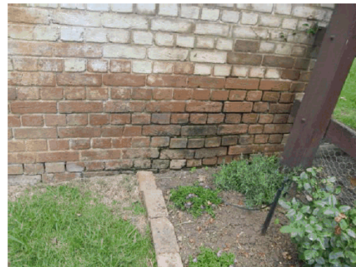
Figure 4.21 View of missing mortar to brickwork adjacent to garden bed and sprinkler.
