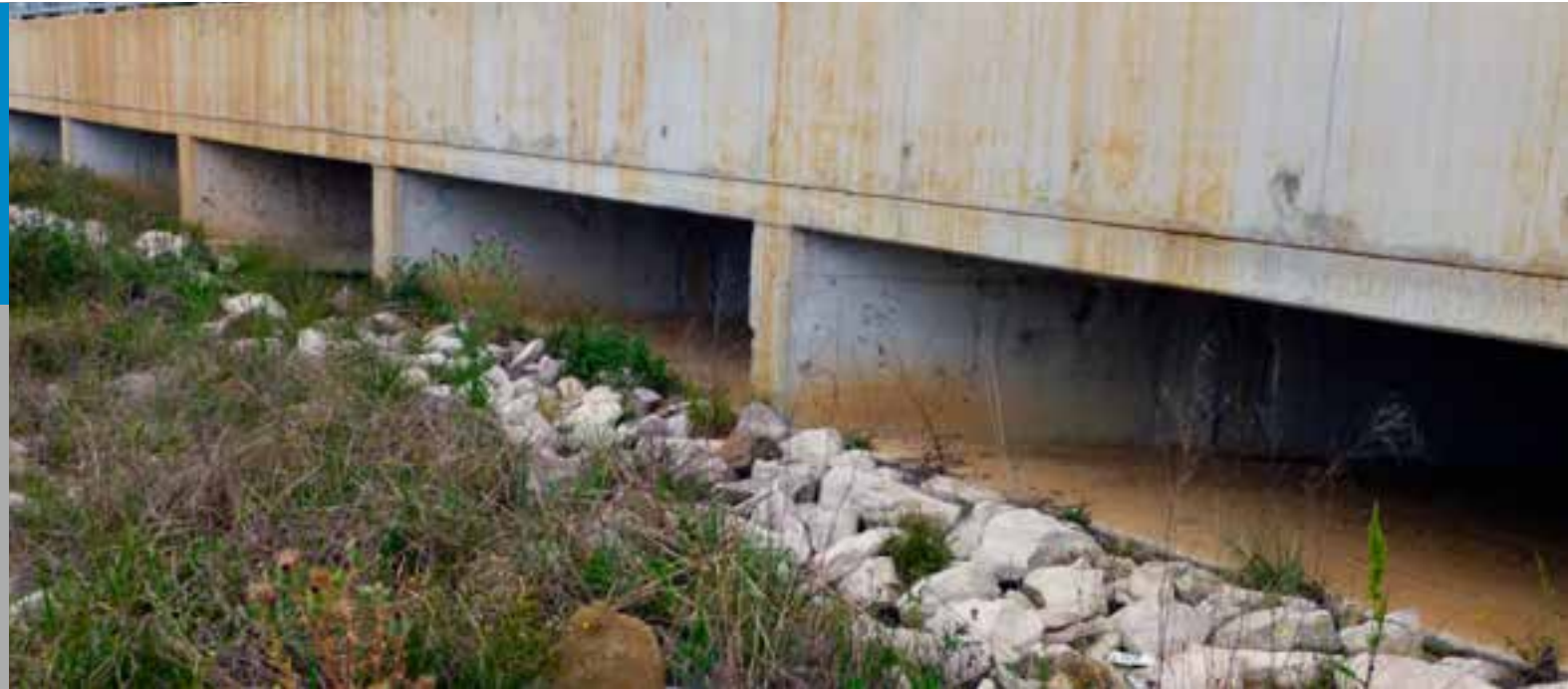
Stormwater Drainage (box culvert) - Liz Kernohan Drive
