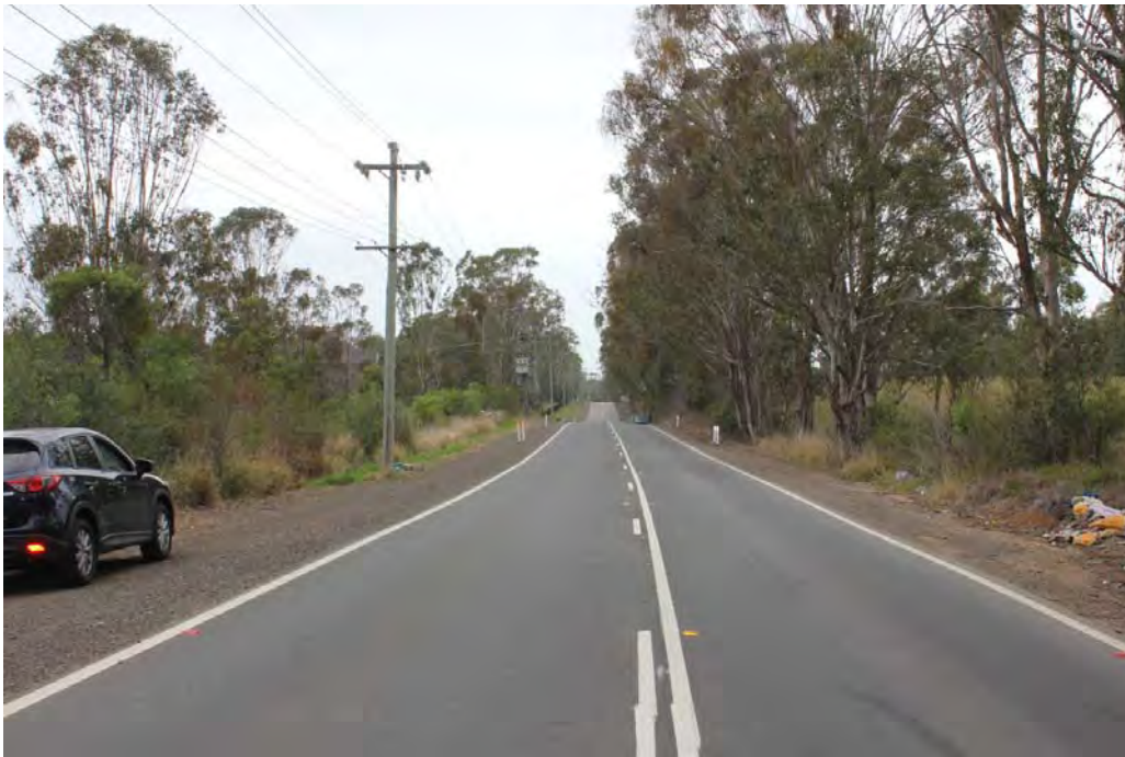
Photograph 2.1 Greendale Road near the proposed site entrance looking east
