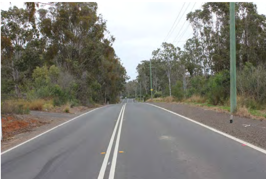
Photograph 2.2 Greendale Road near the proposed site entrance looking west
