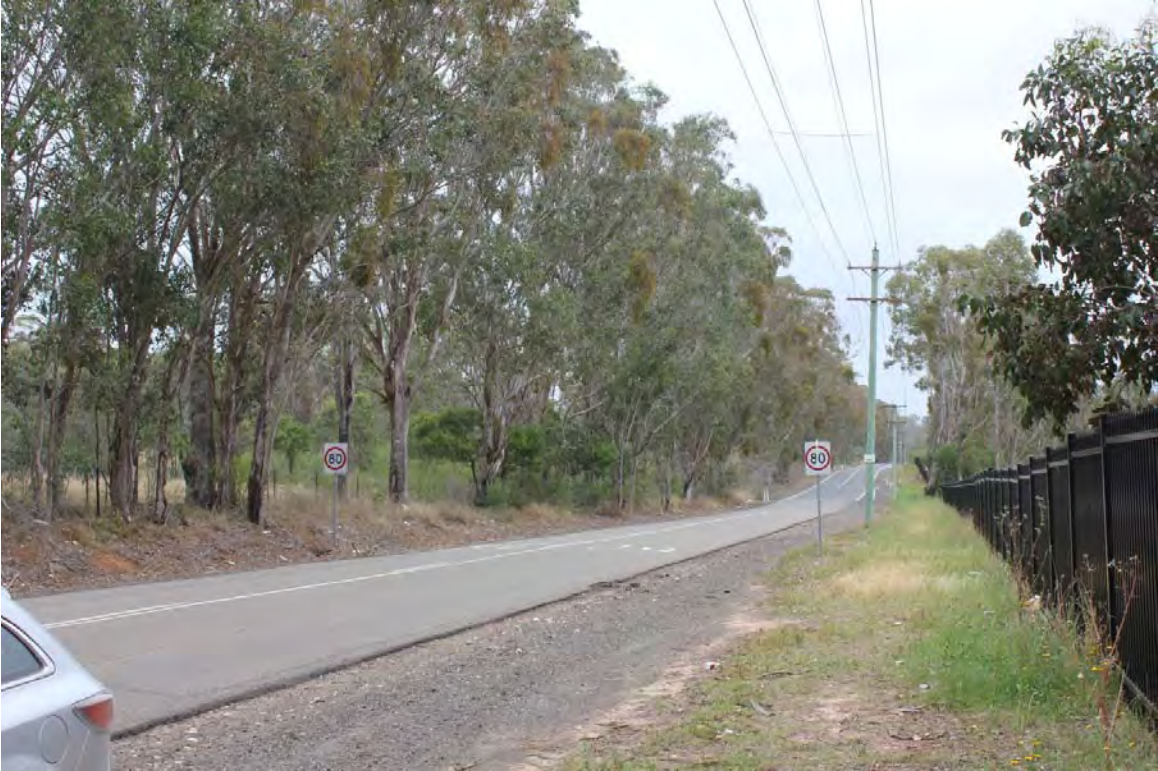
Photograph 2.3 Greendale Road at the speed zone transition point (280 m east of the site entry)
