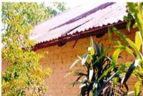
*Image 4.6.* Flaking paint and lifting roof sheets. Facing west. Stedinger Associates 2016.
