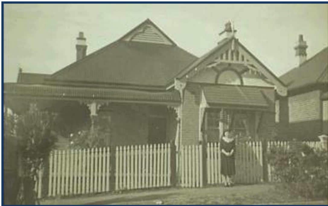
Figure 5: Historical photo of adjoining property at 12 Hill Street from 1920-30s which represents the historical character of the subject property.
