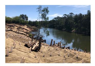
Recent LiDAR measurements show that more than 7,000m³ of sediment was lost from the Ferguson's Land site during May 2022 to July 2023 due to flooding and erosion; that's enough to fill 23,248 bathtubs full of dirt.
