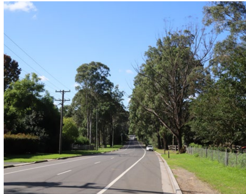
FIGURE 12 VIEW EAST FROM OPPOSITE 365 COBBITTY ROAD
