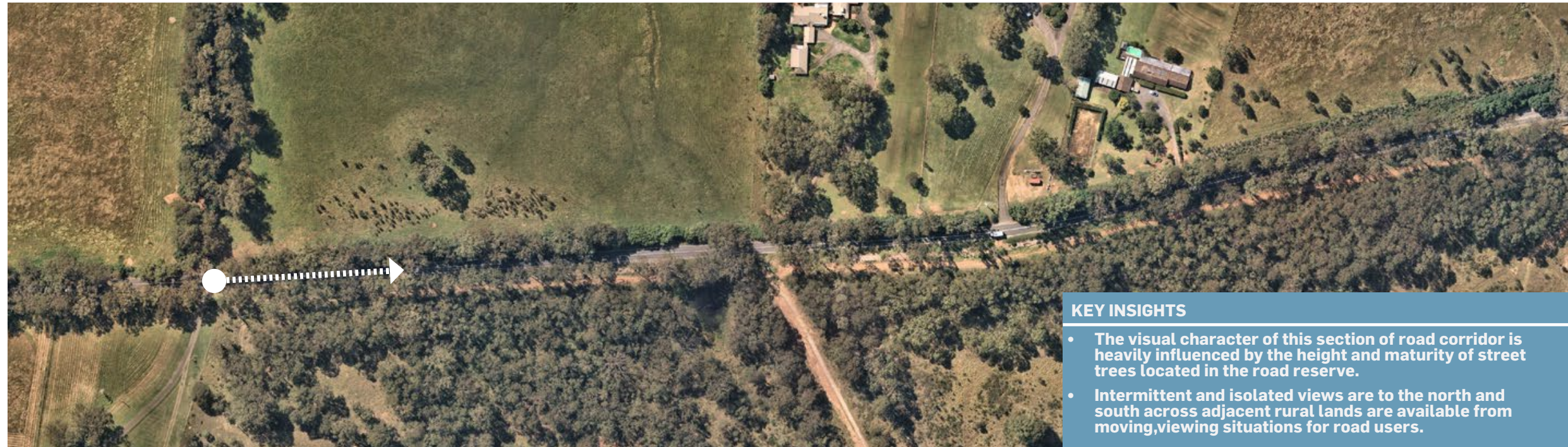
FIGURE 13 ZONE 3 AERIAL AND VIEWPOINT LOCATION
