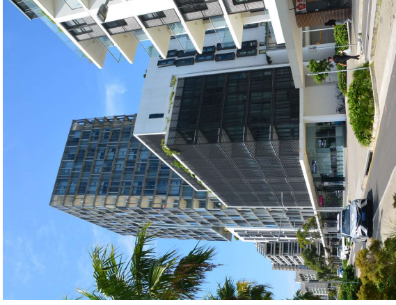
Example of mixed use development with 6 storey street wall with upper levels setbacks to 8 storeys and a 21 storey tower to the corner
