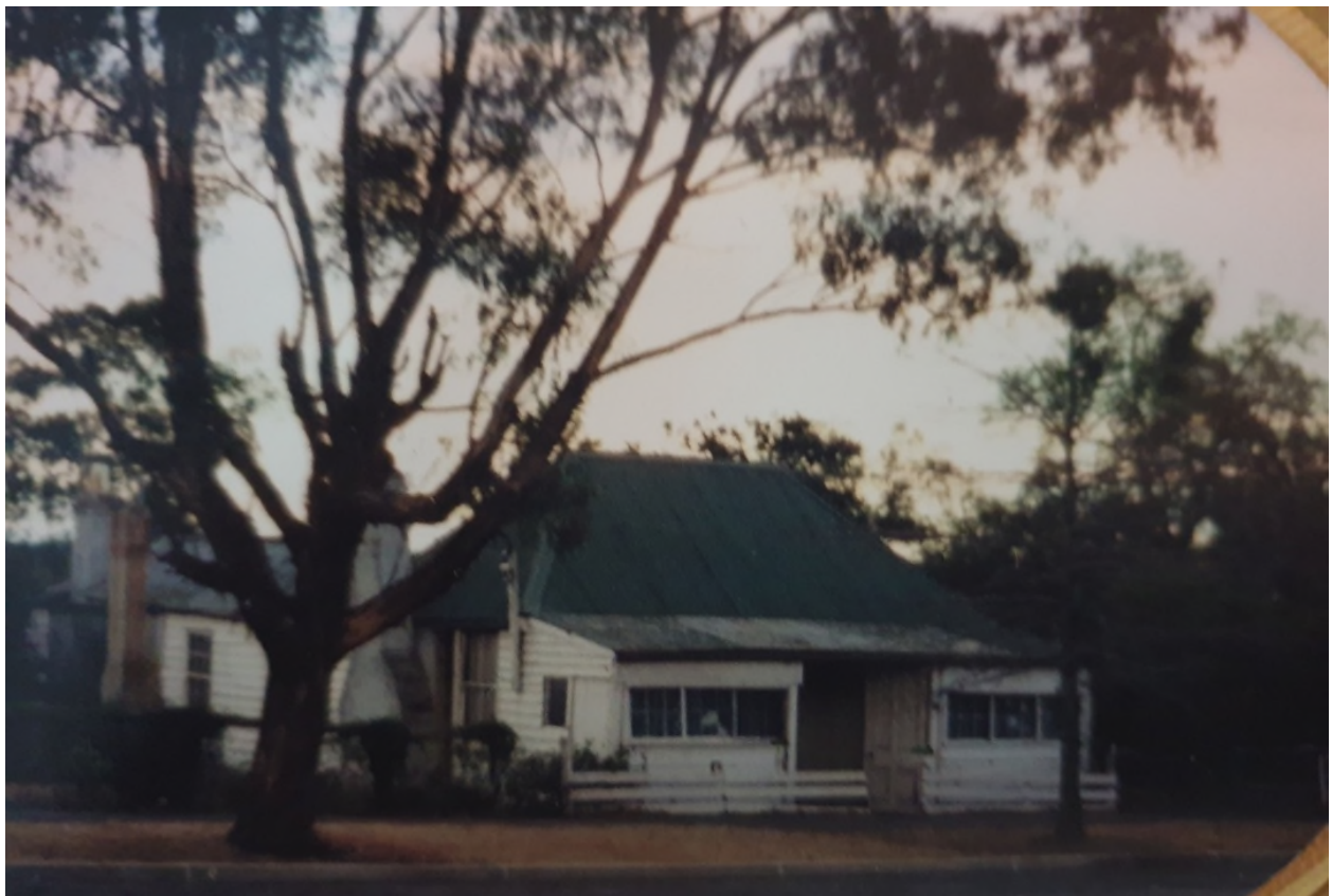
3 John Street, Camden NSW
