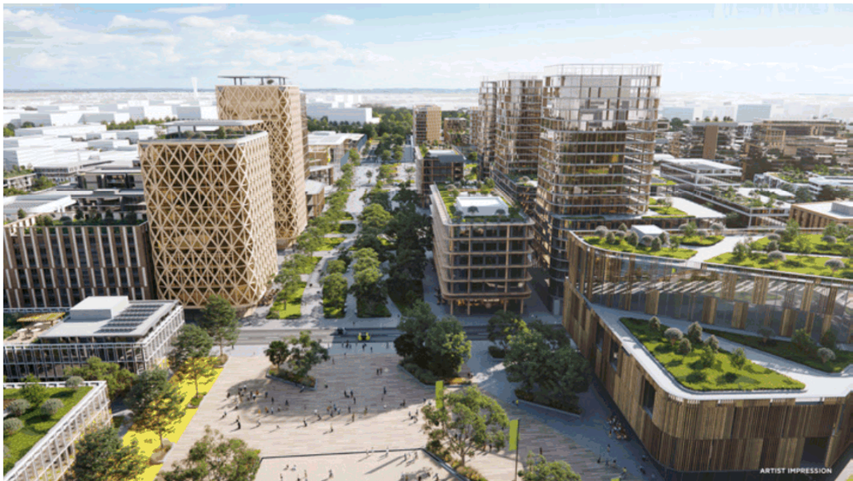
Bradfield City Centre will support a wide range of commercial development opportunities
