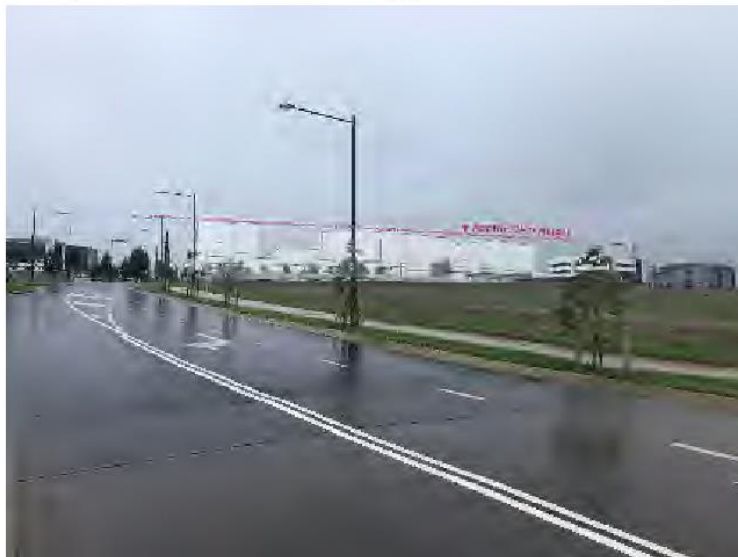
View 4.1 Current LEP Height View - Showing Subject Site DA, reduced to 24m
