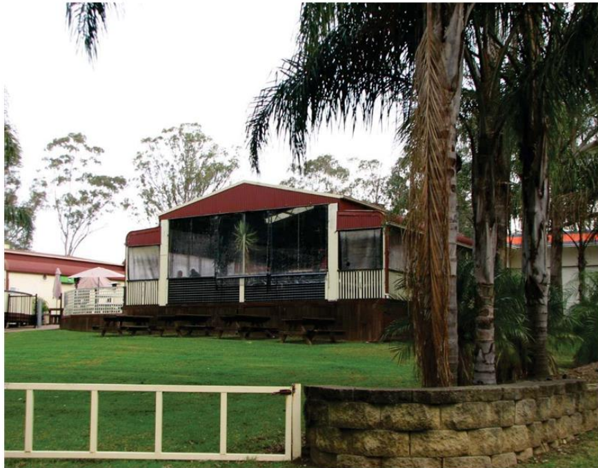
Photo 2: The rear of the existing Lockies Hotel, view east
