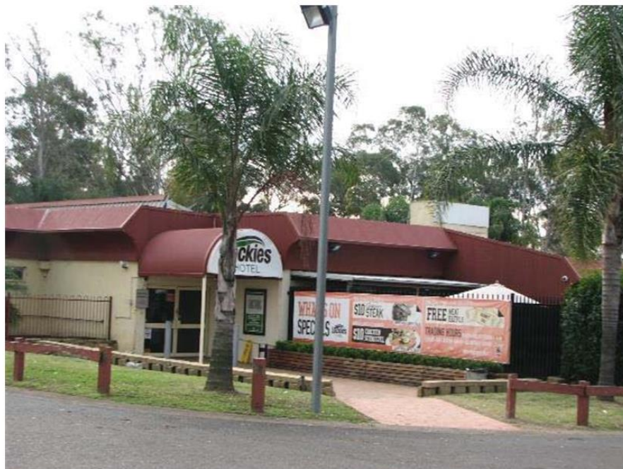
Photo 1: The existing Lockies Hotel, viewfacing north west within site car park
