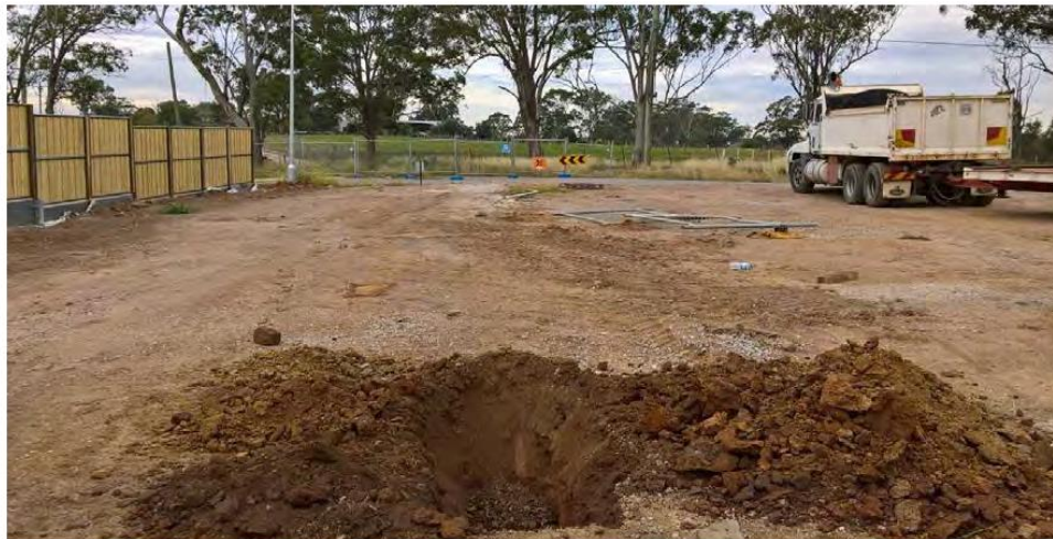
Photograph 10 - Test pit 4 completed in north eastern portion of site.
