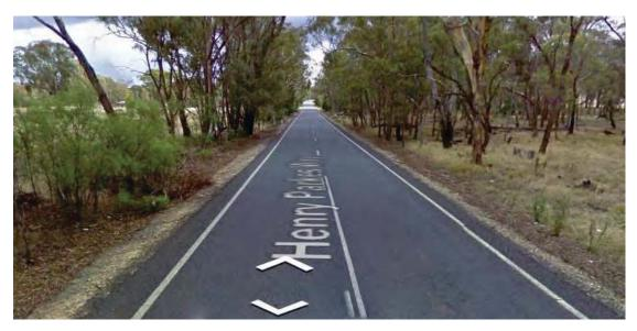
Image caption: An example of a high risk road that lacks safety features to prevent head on and run off road crashes.
