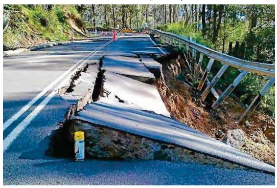
Figure 52: Landslide affecting road infrastructure and traffic movement
