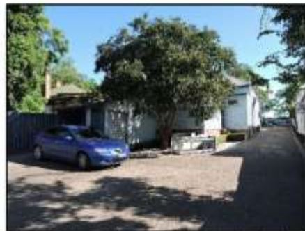
Figure 11. View of the rear of the cottage located on the site. Note the tree and shed addition, which would be removed.
