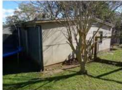
Figure 12: Existing rear garage structure.
