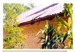
Image 4.6. Flaking paint and lifting roof sheets. Facing west. Stedinger Associates 2016.
