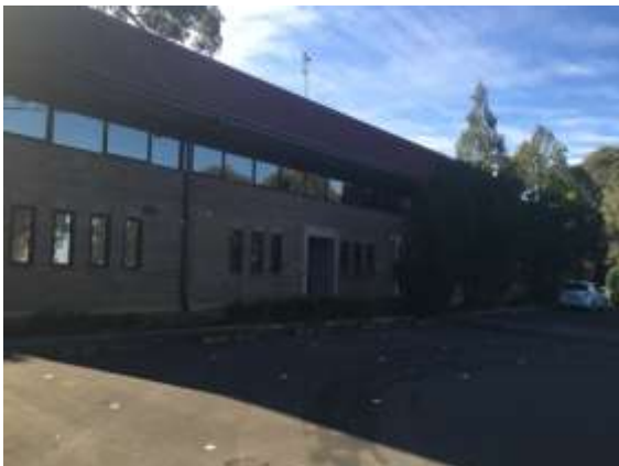
Figure 3 Rear of building taken from the former Council car-park
