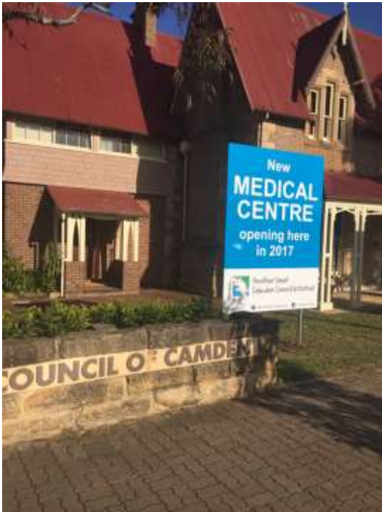
Figure 1 Front of building taken from John Street
