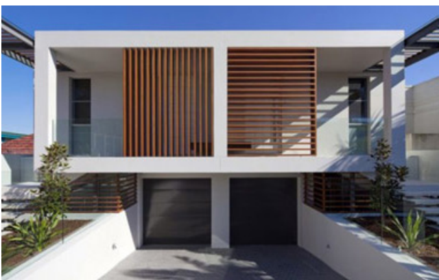
Figure 2-77 Privacy screens can be an integral part of the articulation. Changing the pattern and direction of the screen adds visual interest and asymmetry to the facade
