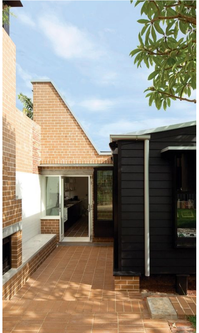
Figure 2-99 Brick patterns create visual interest and add detail and texture. Consider how facade and landscape treatments integrate
