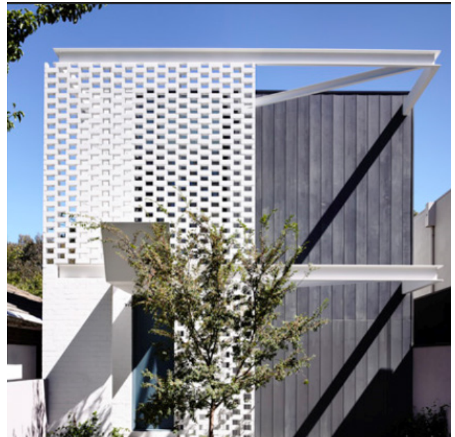
Figure 2-72 Privacy screens are integrated into the facade and provide part of the architectural expression
