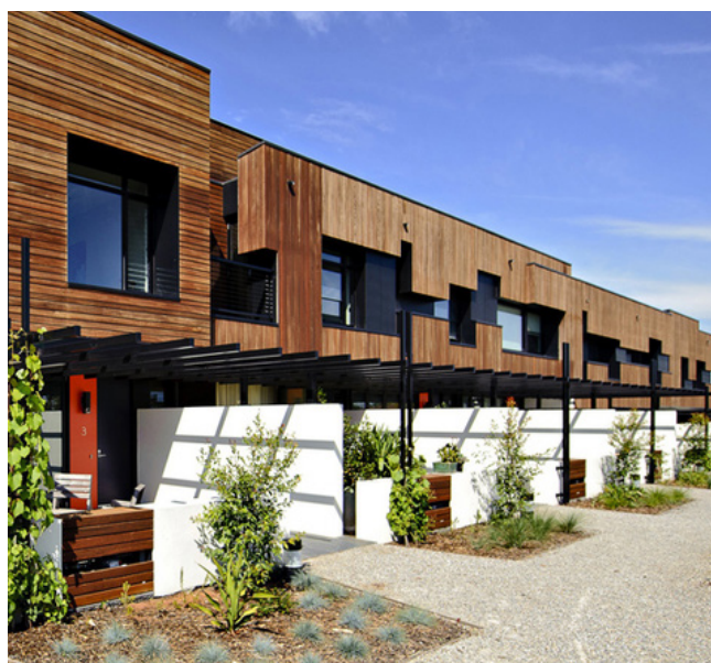
Figure 3-12 Town house development with basement car park
