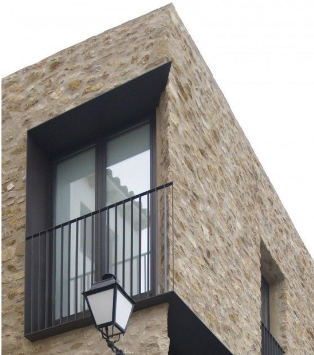
Figure 2-97 Contrast texture with sharply defined openings and fine steel balustrades
