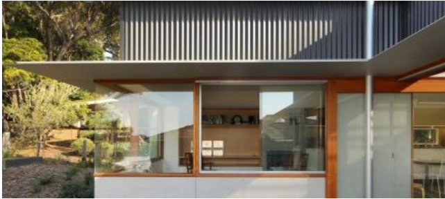
Figure 2-96 Awnings provide shelter and add articulation
