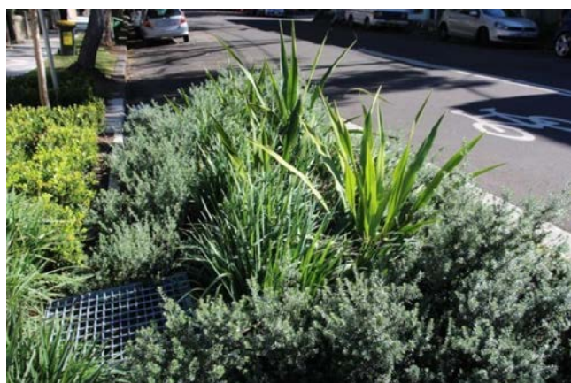
Figure 2-110 Rain gardens integrated into the landscape can filter the stormwater from roads
