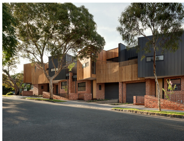
Figure 2-12 Front and rear setbacks provide opportunities for tree planting. Trees should be in scale with the development proposed.
