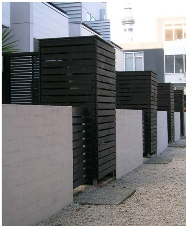
Figure 2-119 Even where bin areas are provided fronting the street they can be designed and incorporated into the building or landscape elements
