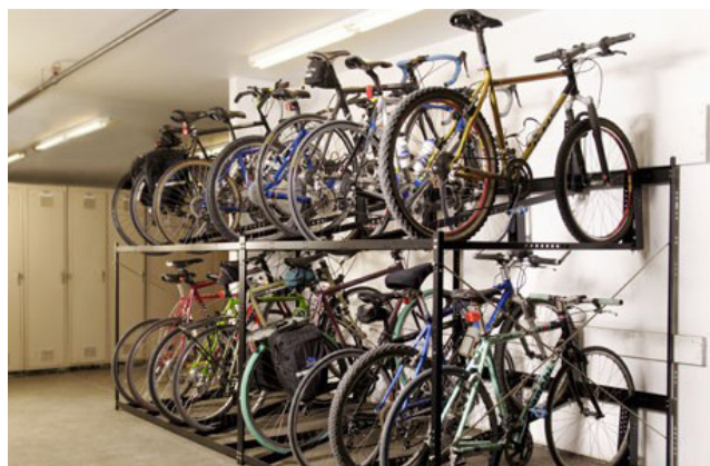
Figure 2-68 Bicycle parking for residents should be secure and easy to access from common areas
