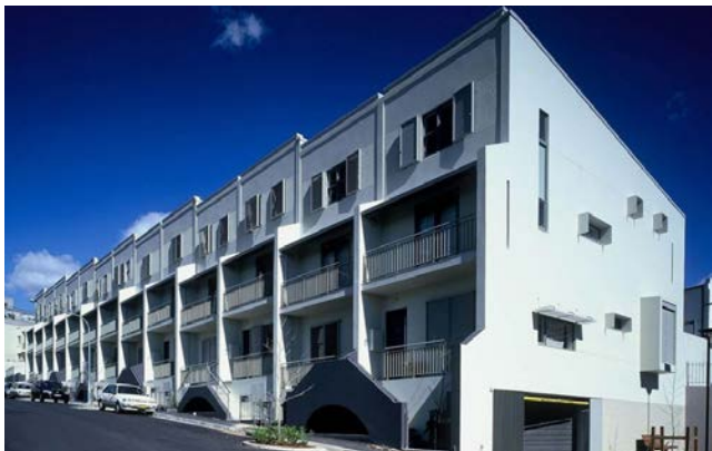
Figure 2-31 Reduce visual impact of basement entries by reducing the scale of the opening
