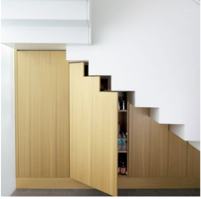
Figure 2-63 Storage space under stairs
