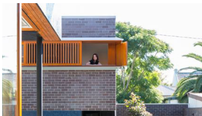
Figure 2-101 Detached studios are separated from the dwelling house. Privacy needs to be considered to avoid overlooking into adjoining properties by restricting inward facing windows and limiting the size of openings to the lane way.
