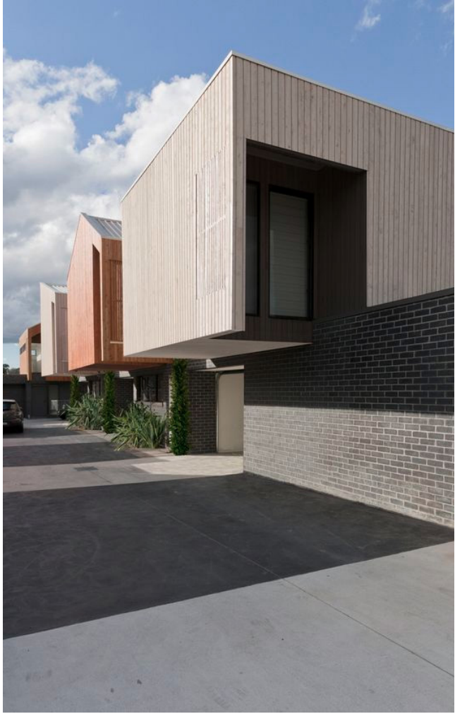
Figure 2-78 A poor acoustic outcome is achieved when driveways are in close proximity to bedrooms and living rooms and driveways are hard paved reverberating sound.
