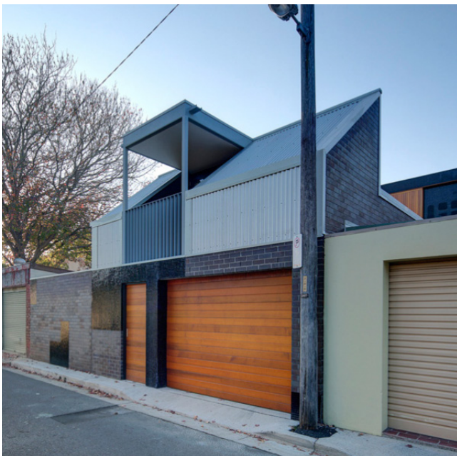
Figure 2-105 Rear outbuildings such as studios should be orientated to the lane to allow for passive surveillance and security
