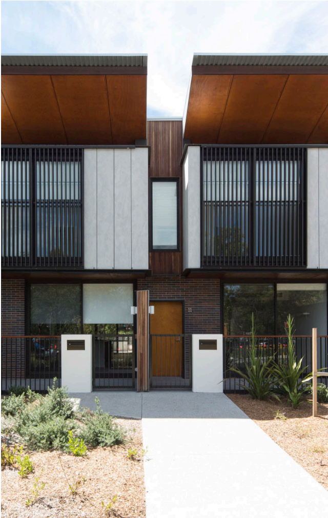
Figure 2-79a Living rooms setback from main circulation spaces by large landscape setback provides privacy
