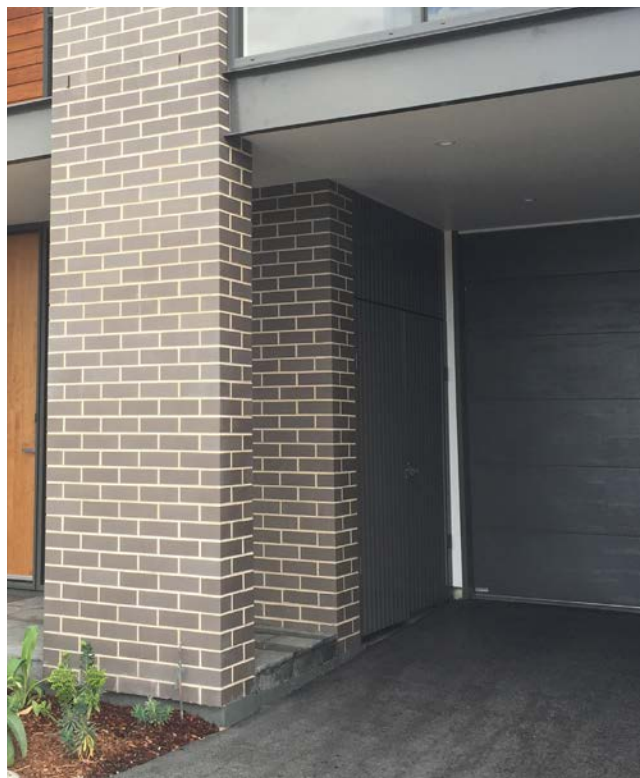
Figure 2-118 Provide bin areas that are screened and incorporated into the landscape or building design
