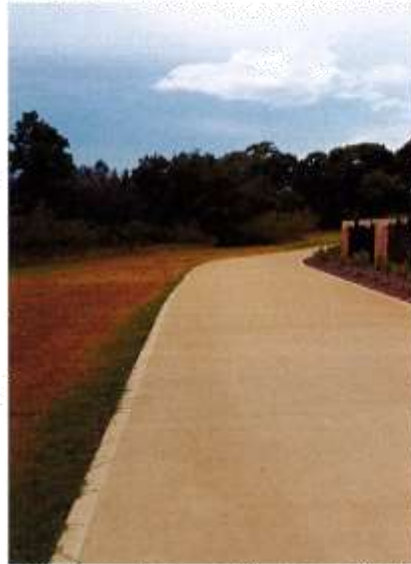
Existing Pathway Location B
