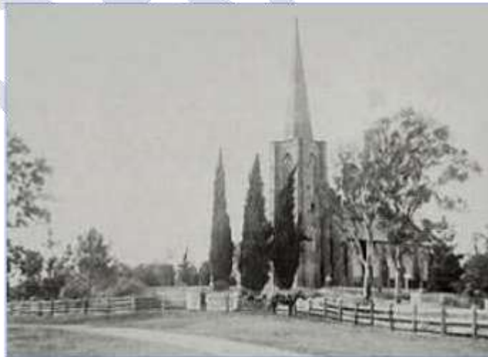
Figure A – A photograph of St John's Anglican Church, Camden taken by 1896 shows that a pair of Forest Red Gums ( Eucalyptus tereticornis ) (right), remnants of the original woodland, were large specimens even at this time. The same trees are still thriving on the
