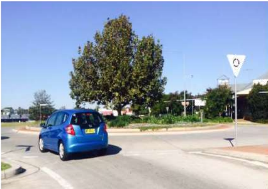
12. Roundabout at Holdsworth Drive and Main Street, Mount Annan
