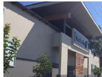
Variations to the wall facade including protruding elements which should be encouraged along the riparian interface particularly where visible from the public domain and key pedestrian cycle links.
