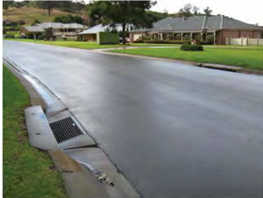
Photo 5: Typical Road Drainage
