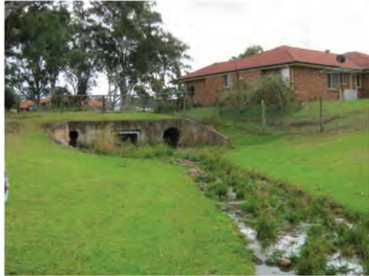
Photo 9: Headwall With Culverts Discharging Downstream of The Meadows
