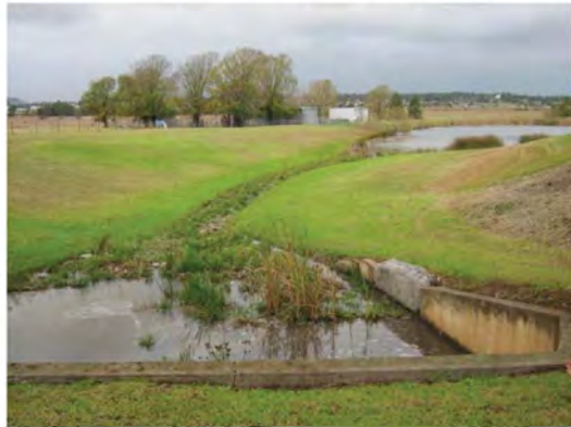
Photo 10: Existing Channel and Dam Downstream of The Meadows
