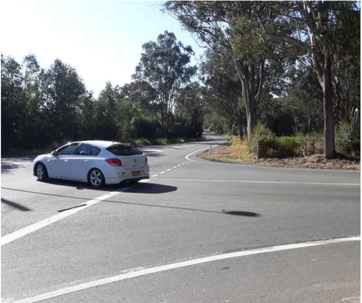
Figure 2.10: Cobbitty Road at Macquarie Grove Road (looking east)
