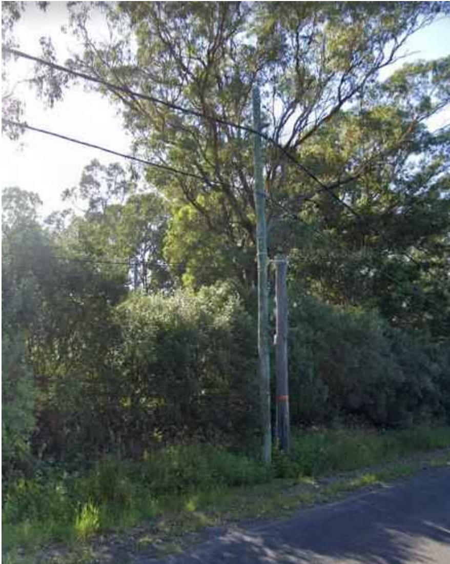
Figure 2.9: Utility Poles in Kirkham Lane
