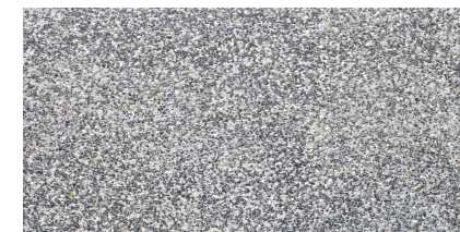
6. EXPOSED AGGREGATE CONCRETE (DRIVEWAY)
