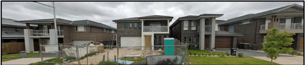
Figure 2: 6 Dustan Street and development adjacent the subject site (Google Streetview)
