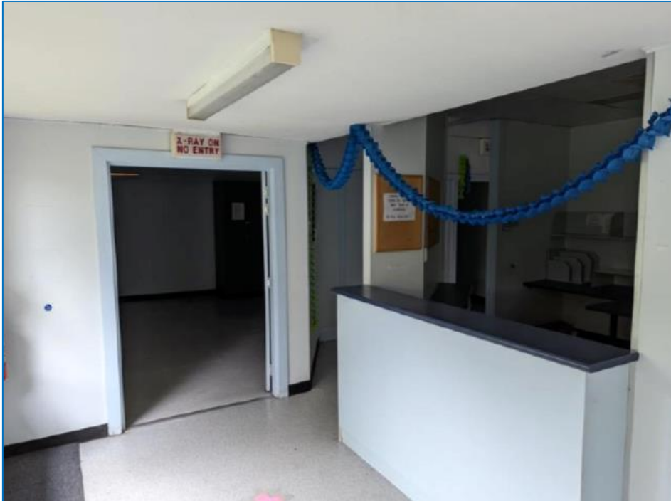
Figure 13: Internal alterations / fit-out for commercial use (formerly X-Ray Clinic).
