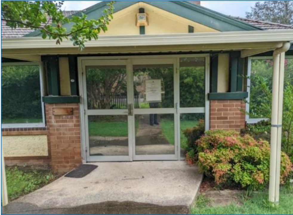
Figure 11: Inserted aluminium framed door to primary eastern elevation.
