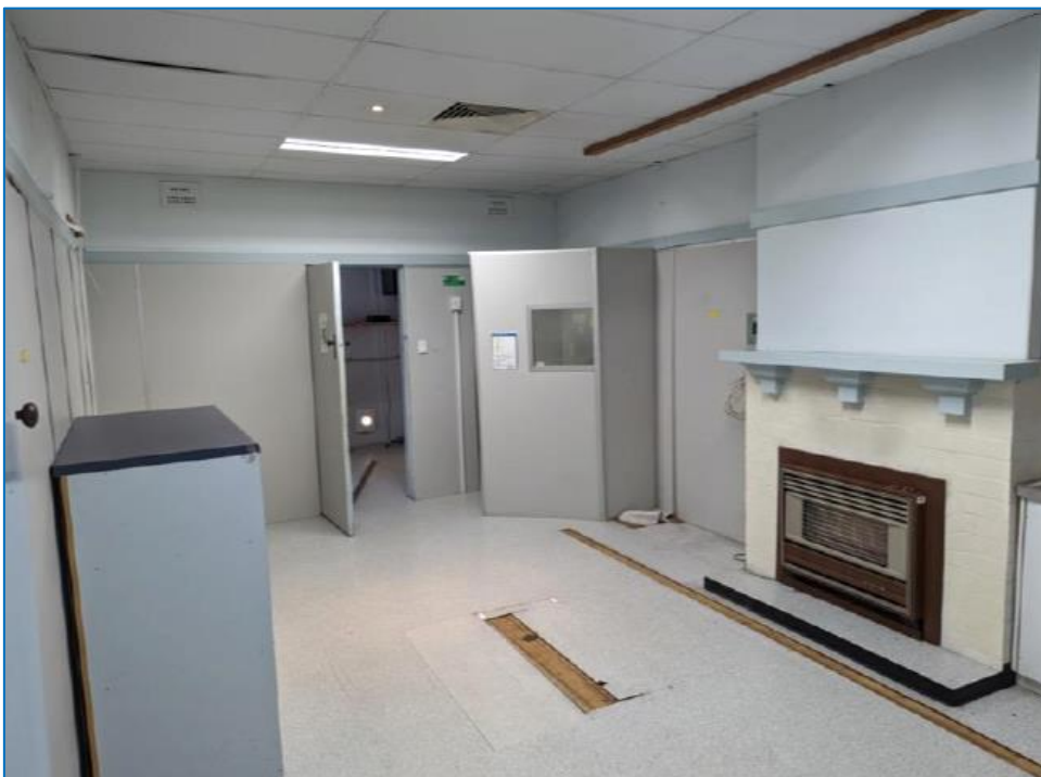
Figure 14: Internal alterations / fit-out for commercial use (formerly X-Ray Clinic).
