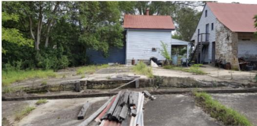
Image 1 – General view of the site, showing the 2 floor layers (1929 and 1970)
